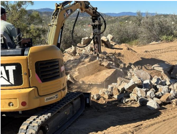
Breaking up the pads
