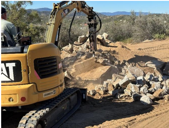
Breaking up the pads
