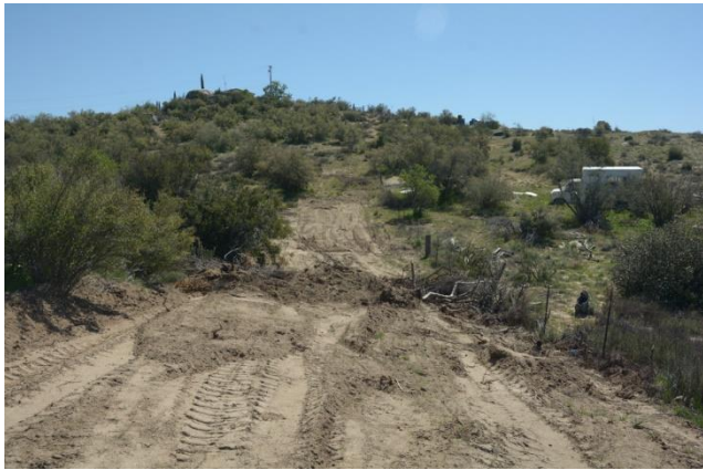
East view along SouthBreak
