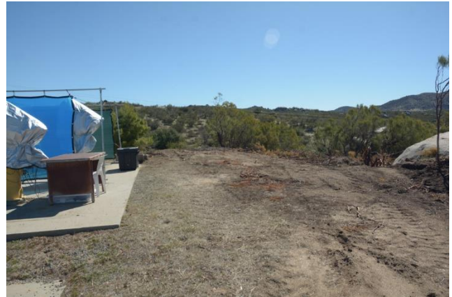
Upper Pads clear-out along its southern edge looking east
