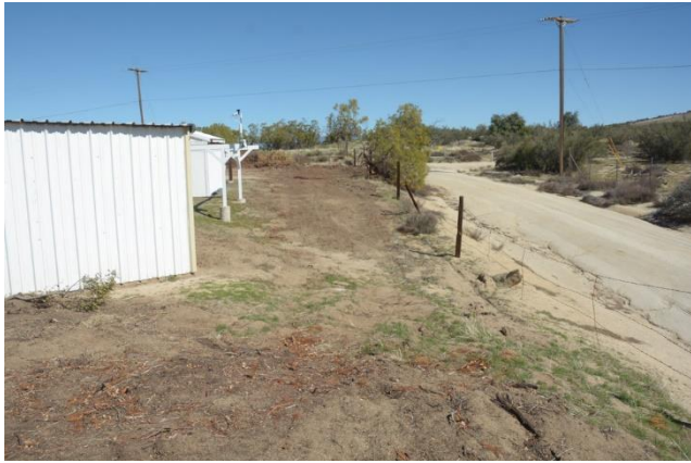
North view of northeast corner of site at Upper Pads
