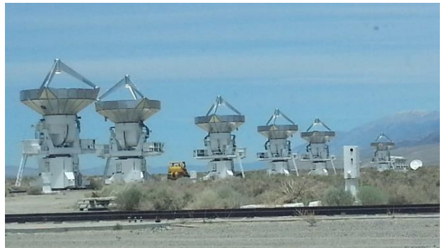
Ex Carma Array dishes at the site.
